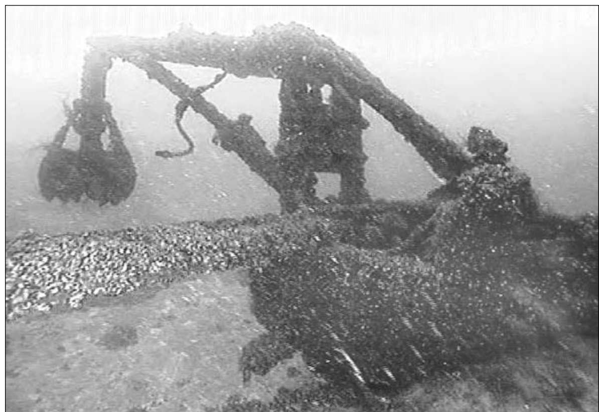
Moving with the Lake Huron current, a cable still dangles from the arm of the clam bucket scoop attached to a work barge that sank around 1947 between St. Ignace and Mackinac Island. This underwater picture was taken from a film of the wreck Wednesday, August 5. Crew aboard the Pride of Michigan used a remote operating vehicle to film and explore the site. Information about the barge will be given to state archaeologists, who will research and document the find. (Photograph courtesy of Luke Clyburn)
